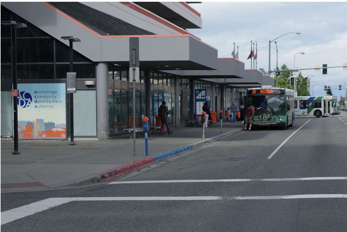
Figure 1: Photograph of the Existing Transit Center on West 6th Avenue from G Street during a weekday.
